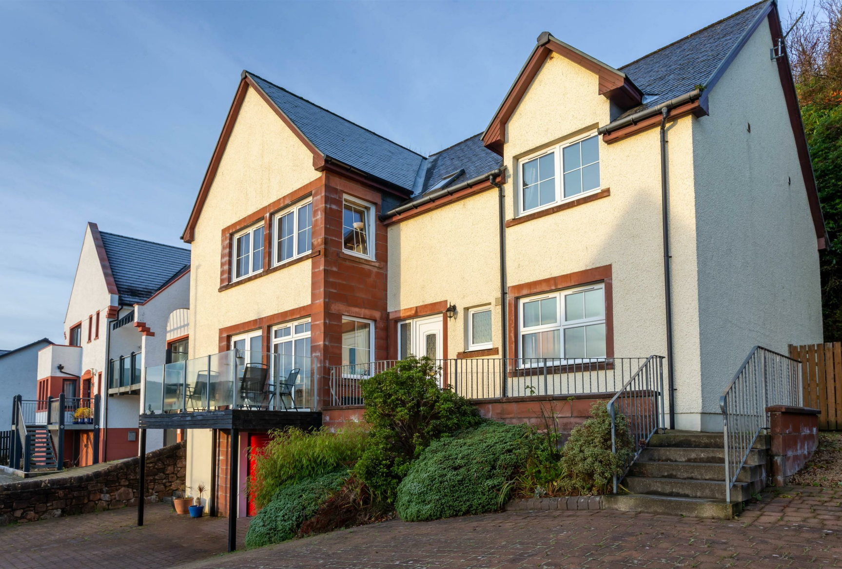
Stonewater House, Shore Road, Lamlash, Isle Of Arran, KA27 8JN
